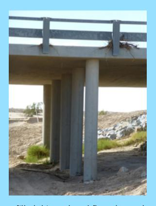
water filled this wash and flowed over the bridge. Debris is seen on the downstream side of the SB lanes of Hwy 86 in the guard rails.
